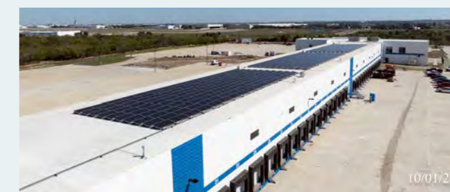
Solar panel installation at our new site in Haslet, Texas
