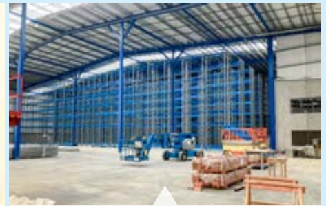
New racking being installed (15,000 pallets)
